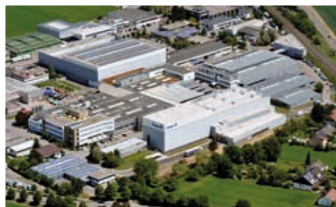
Left: The Ensinger company headquarters in Nufringen near Stuttgart. Home to the company's administration, production and warehousing activities.
